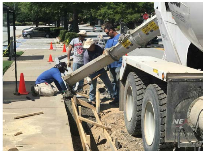
Form, place and finish remaining concrete, 9.16
