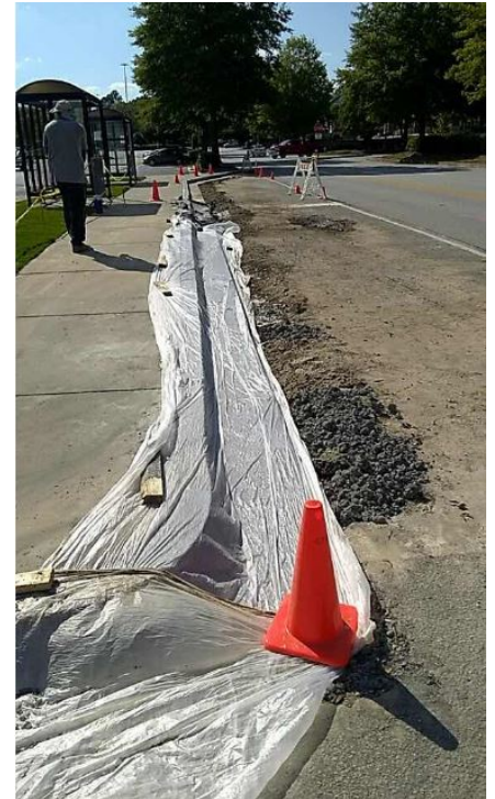
Protect newly placed concrete
