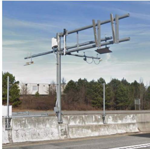
Figure 1 Example of overhead gantry along the I-85 Express Lanes and Extension projects
